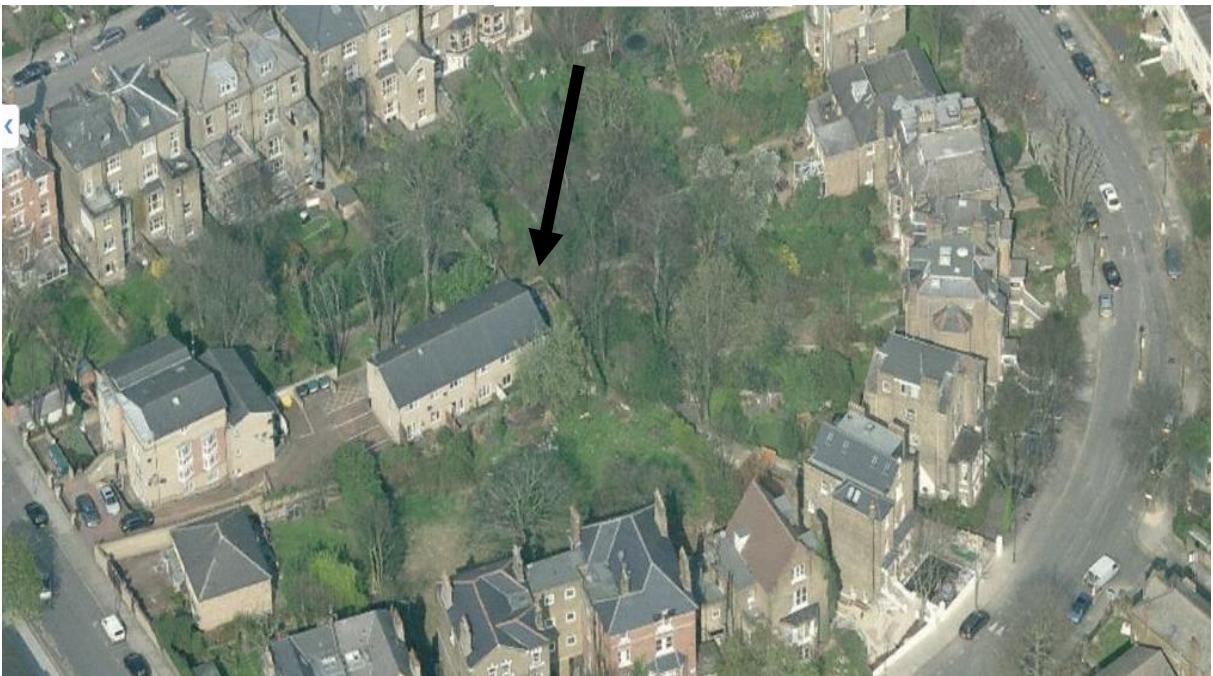
Image 1: Aerial photograph showing the rear garden of 55 Carleton Road.
